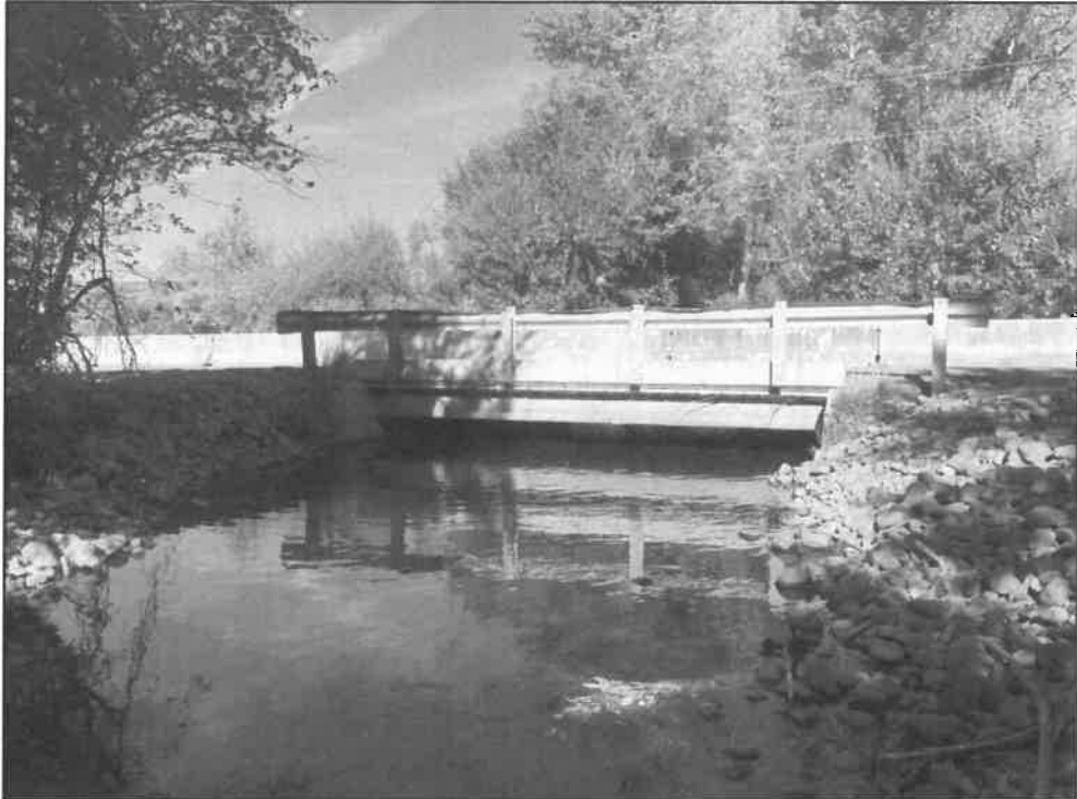
Photo 3. Bar 14 Road Bridge from downstream.
